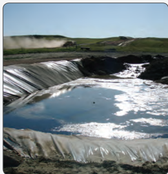
“Mud pit” on a Bakken shale drilling site.
